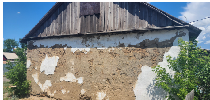
Fig. 4. An example of a mudbrick barrack which was converted into a house after Karlag closed.
